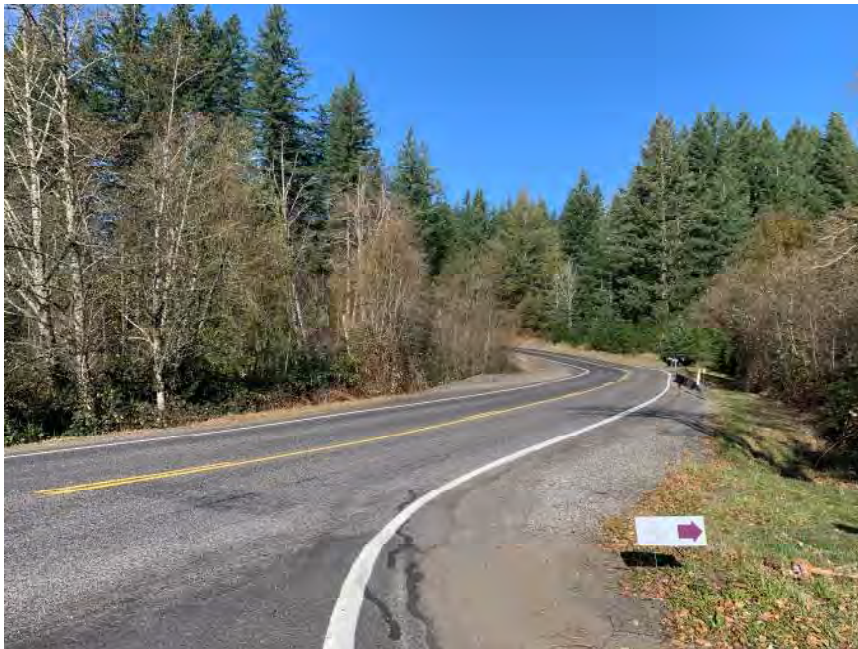
Figure 4: Example of Pavement Markings
