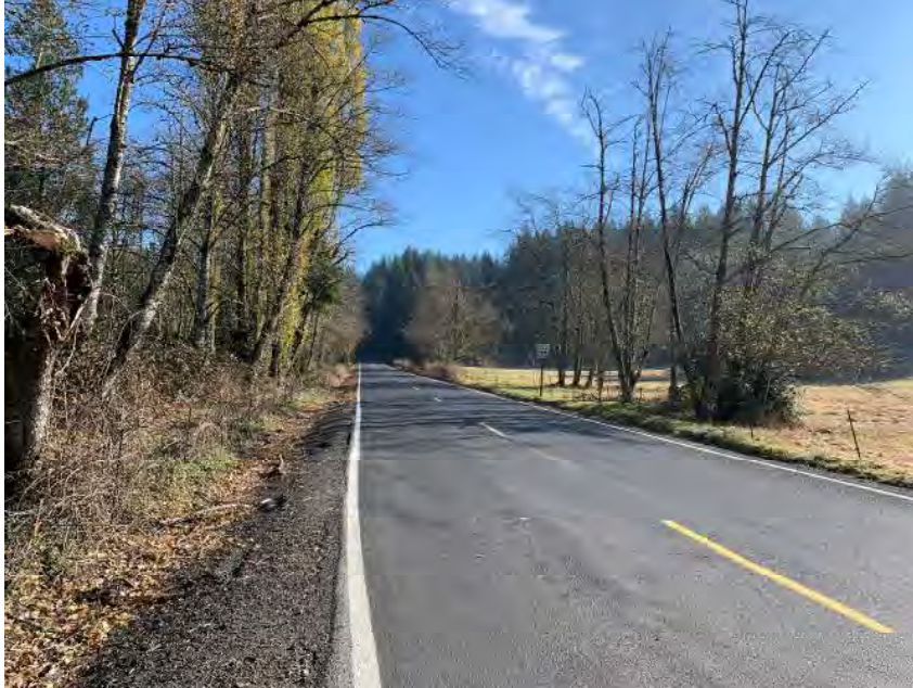
Figure 3: Example of Pavement Markings
