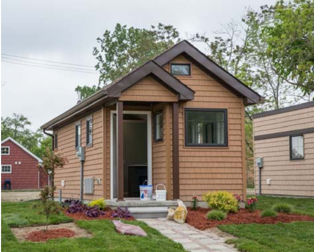
A site built dwelling meeting building code (allowed in Skamania County)
